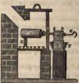
The figure in the margin reposed a section of the furnace, with a iron bottle A, supported by the brick B. To the mouth of the bottle a short iron tube C, (a per of a gun barrel will answed) either to be fitted by means a female screw in the mouth of bottle, or simply by grinding. It tube must pass through a hole if fire-brick, with which the mouth
